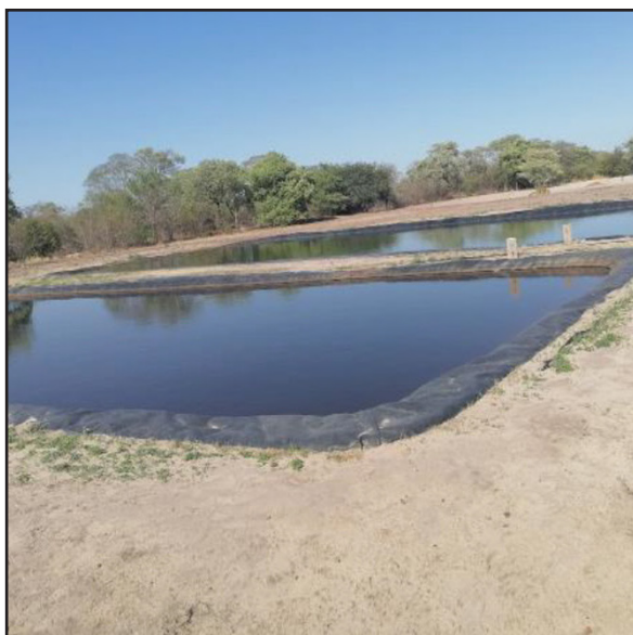
a) Earthen pond
