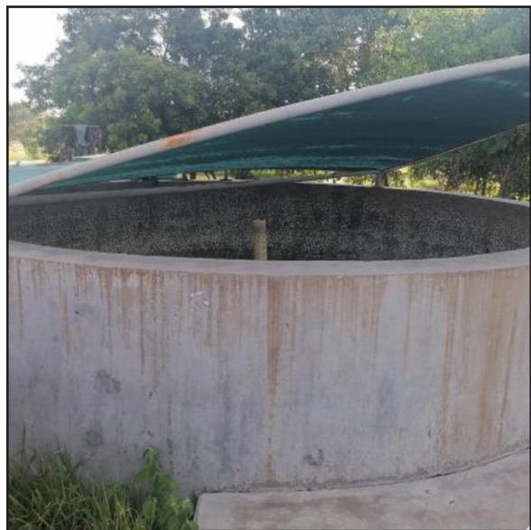
a) Earthen pond
